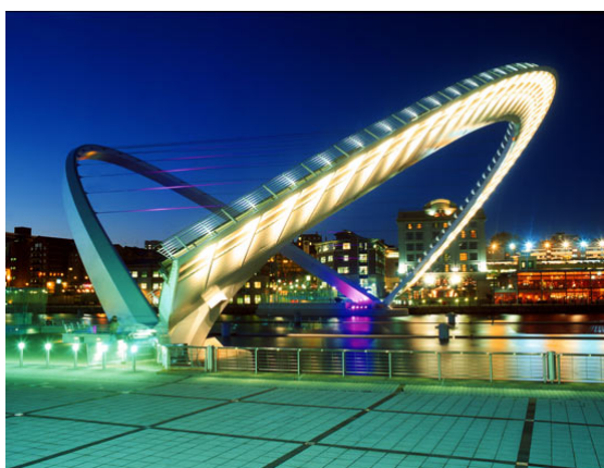
Gateshead Millennium Bridge
